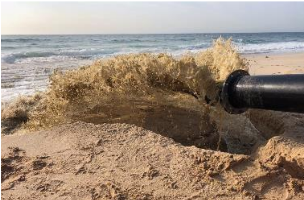
Photo 9: Dredged sand deposition showing energy dissipation via deflector plate
